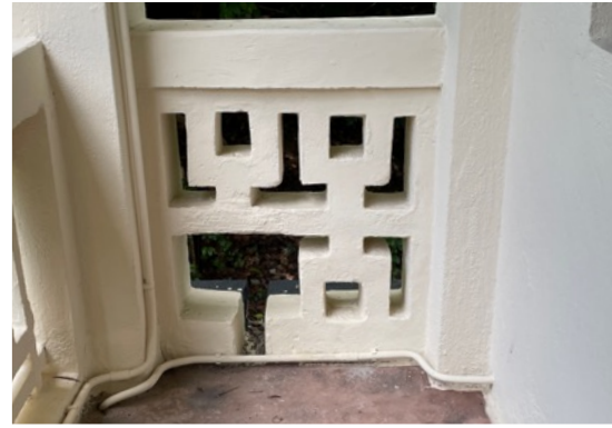
Figure 80 Pattern balustrades of longevity symbol with drain outlet in 2023.
